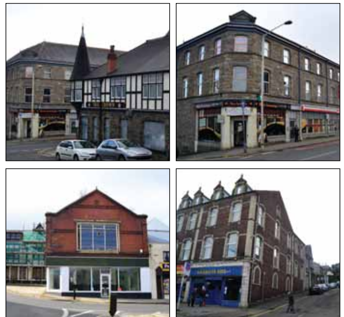
Figure 30: Examples of strong corner buildings
